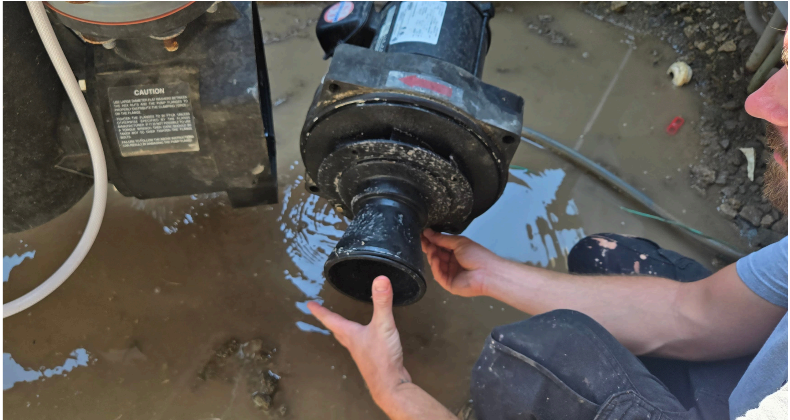
HARRY MYERS POOL: PUMP REBUILD
